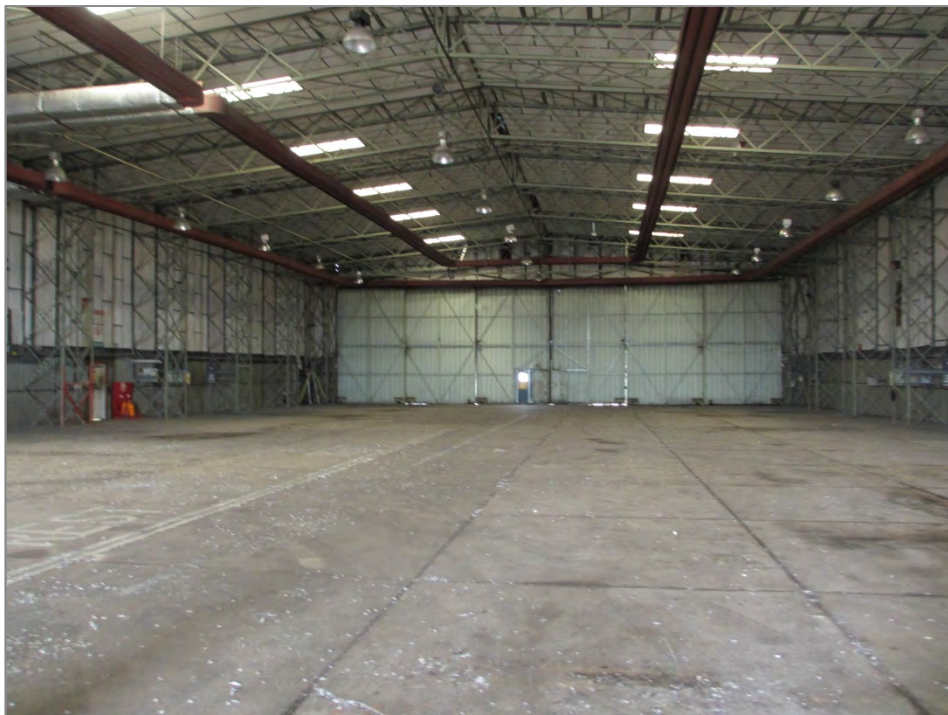
Figure 18: First cargo hangar interior
