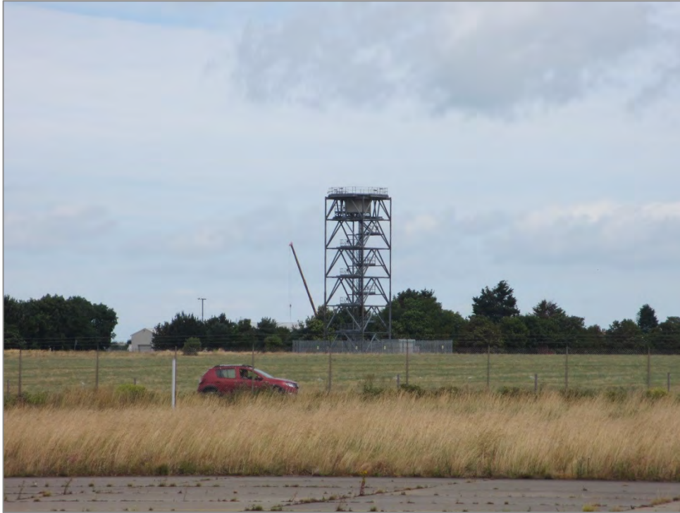
Figure 12: Radar tower with radar removed
