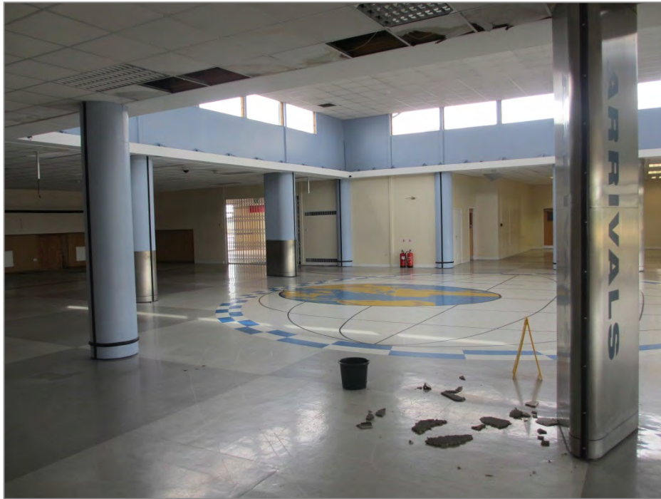
Figure 3: Main foyer of terminal building from arrivals. Check-in area to the left of the image.
