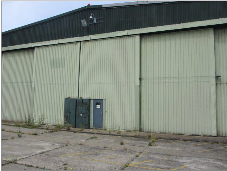
Figure 17: First cargo hangar exterior
