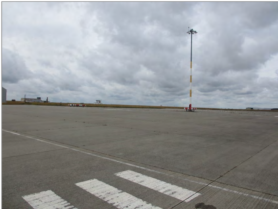
Figure 6: Apron as viewed from terminal
