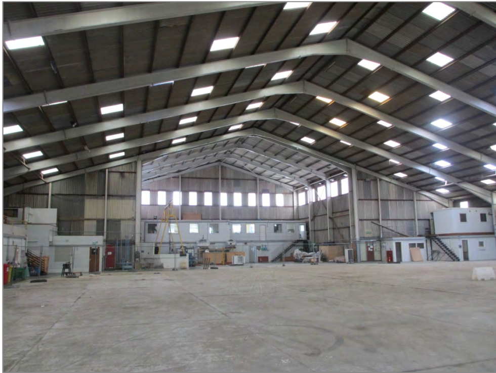
Figure 15: Interior of maintenance hangar
