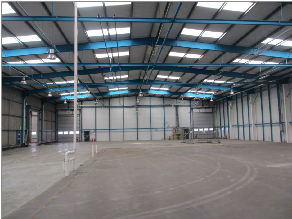
Figure 20: Second cargo hangar interior
