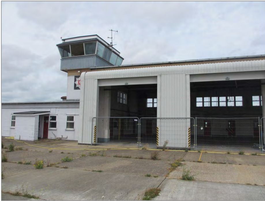
Figure 13: Dilapidated Rescue & Fire Fighting Facility
